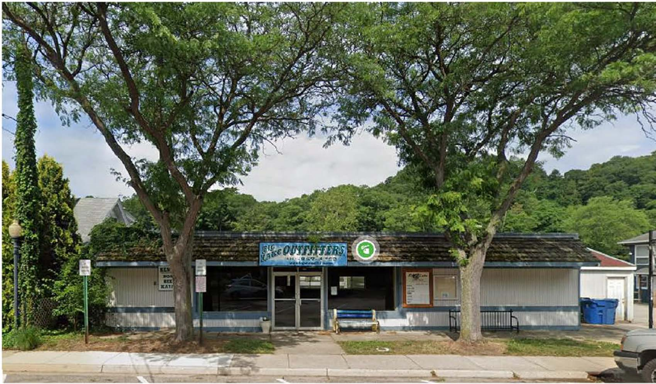
PHOTO OF EXISTING BUILDING TO BE DEMOLISHED
