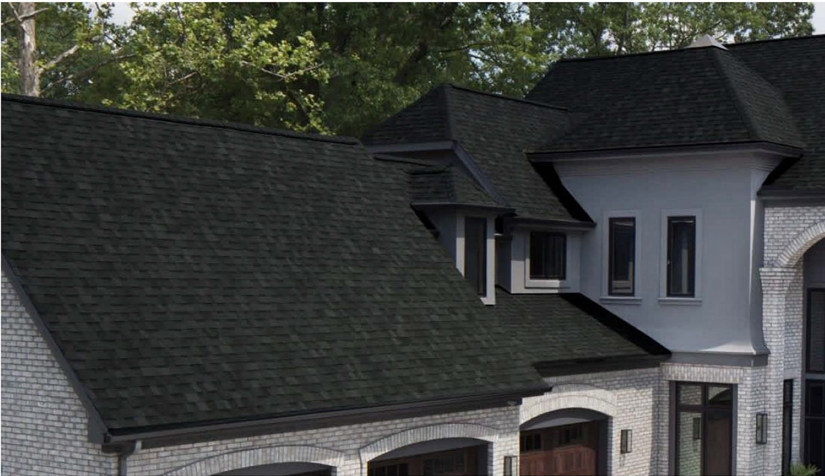
Example image of roof shingles.
