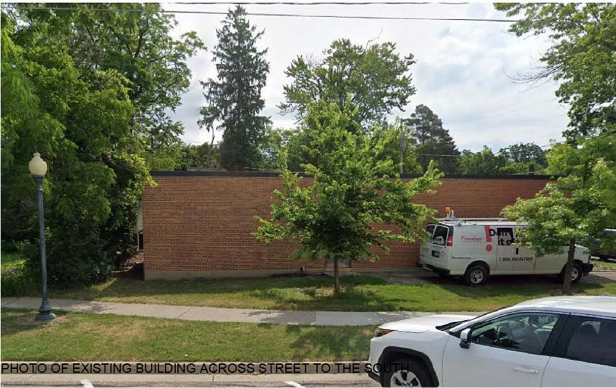
PHOTO OF EXISTING BUILDING ACROSS STREET TO THE SOUTH
