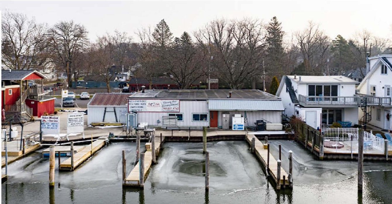
PHOTO OF EXISTING BUILDING TO BE DEMOLISHED ON RIVER SIDE
