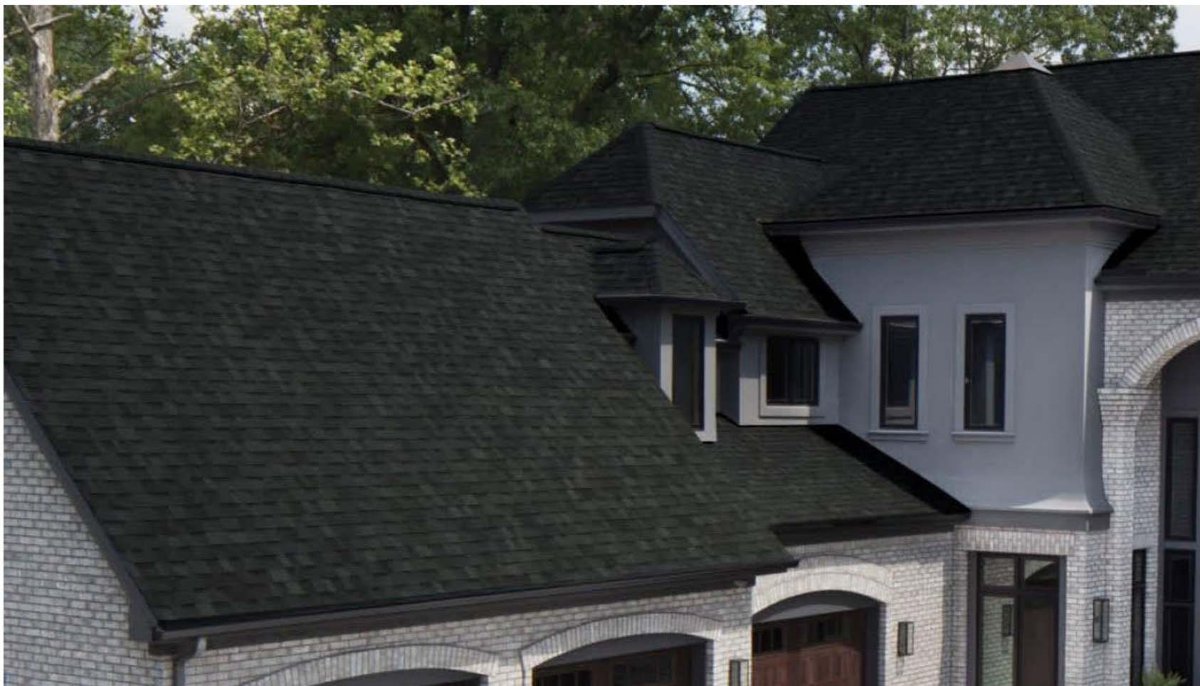
Example image of roof shingles.
