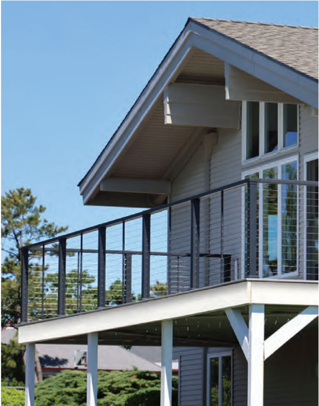
Example image of cable guardrails.
