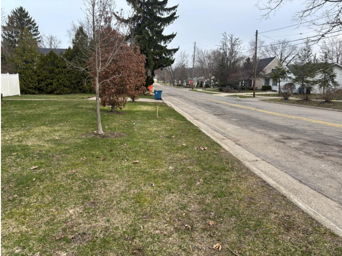
Sidewalk Extension – North of Mason Street, facing north, along 580 Mason Street
