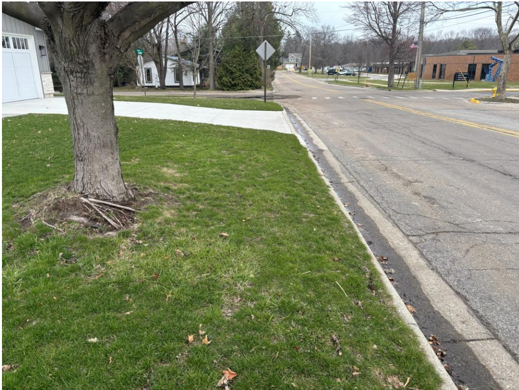
Sidewalk Extension – 330 Elizabeth Street, facing north, tree impact
