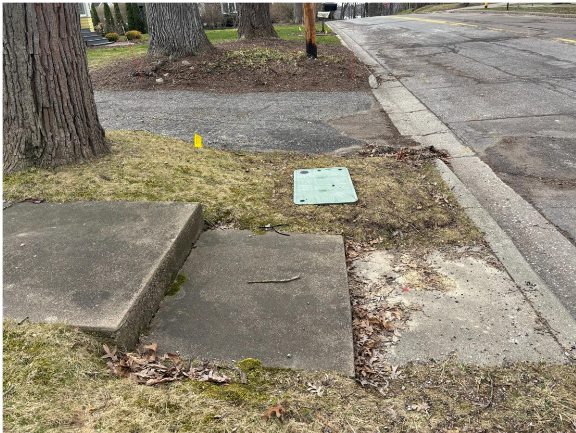
Sidewalk Extension – 165 Elizabeth Street, facing south
