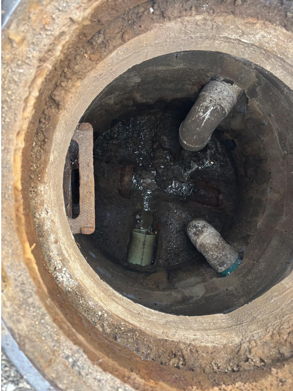
Sanitary Manhole SS1475 – Photo 2, internal drop connections
