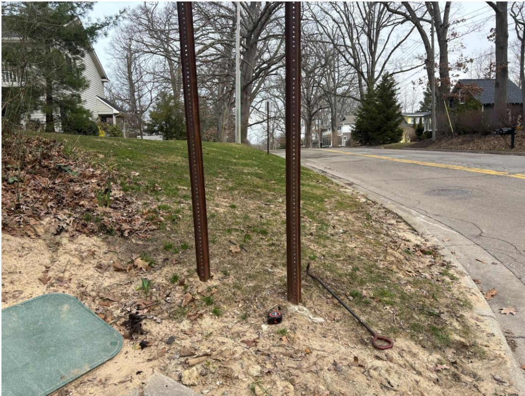
Sidewalk Extension – 124 Elizabeth Street, facing north
