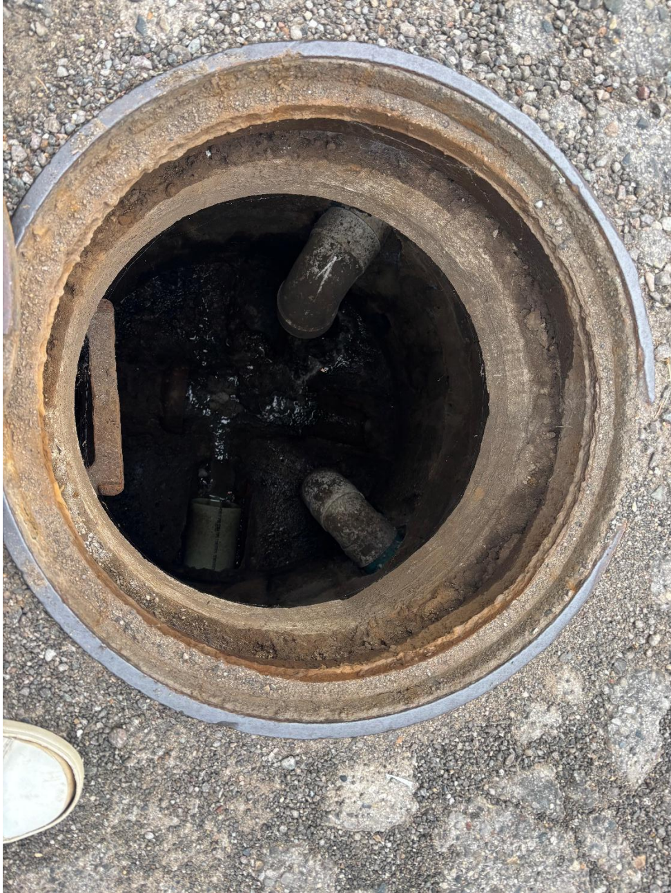
Sanitary Manhole SS1475 – Photo 1, internal drop connections
