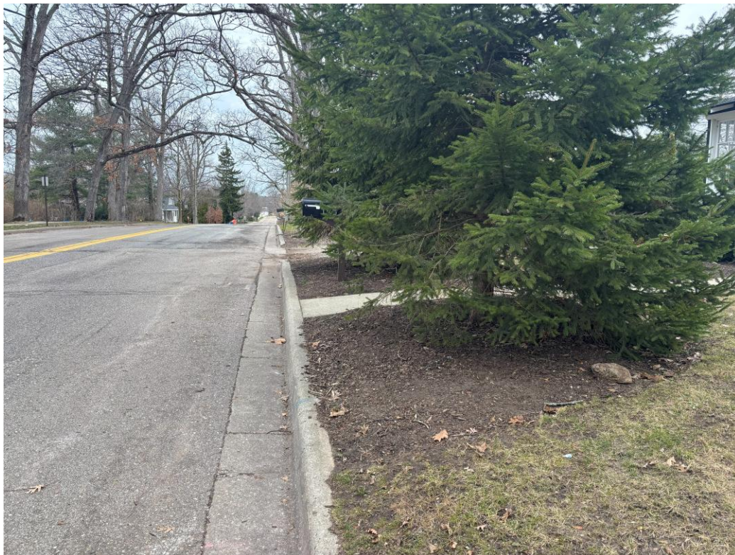
Sidewalk Extension – 125 Elizabeth Street, facing north
