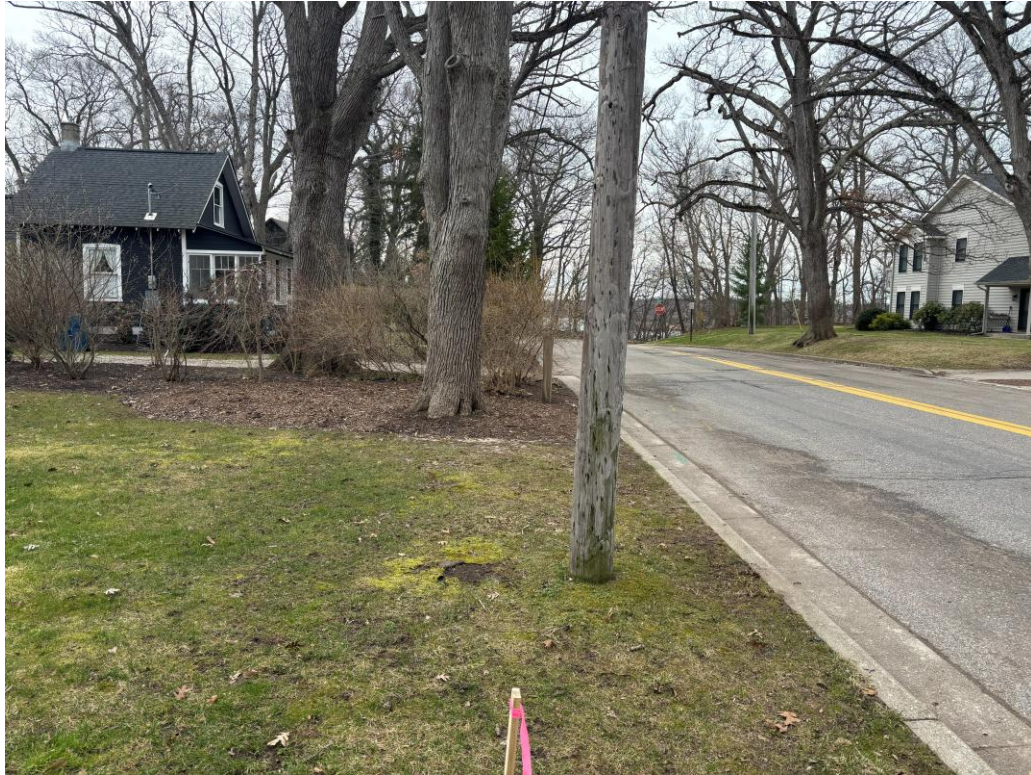
Sidewalk Extension – 143 Elizabeth Street, facing south
