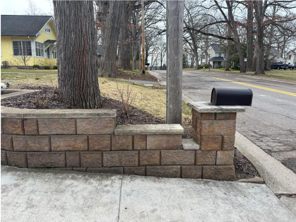
Sidewalk Extension – 165 Elizabeth Street, facing south
