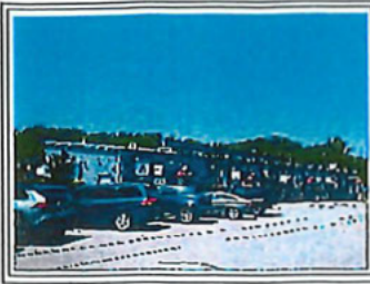
VIEW OF THE FRONT OF THE SUBJECT LOOKING NORTHERLY
