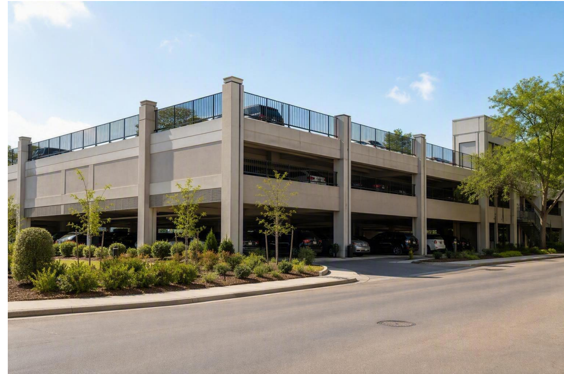
Illustrative example: three-level parking deck, Rochester Hills, Michigan.
