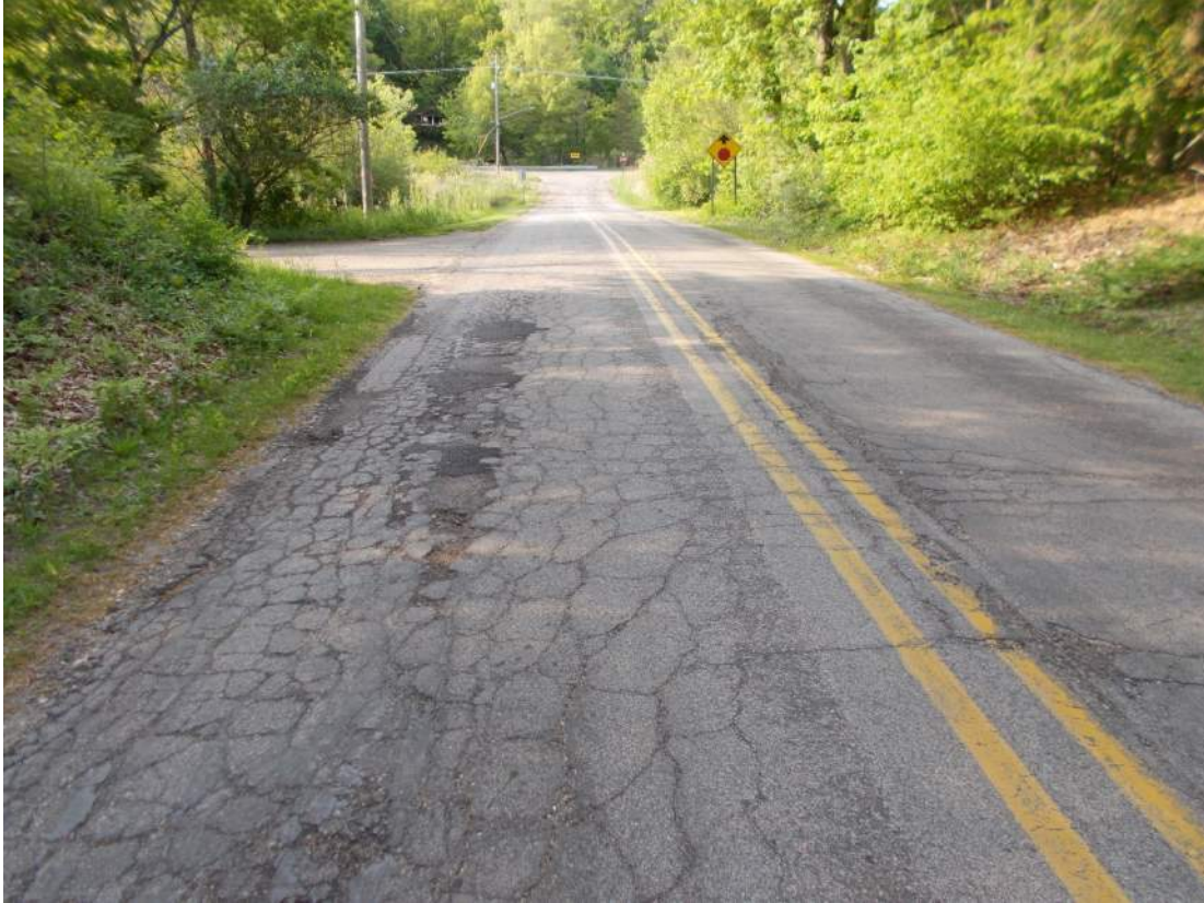
Maple Street looking north toward North Street
